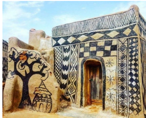
Traditional earthen architecture in the village of Tiébélé, Burkina Faso.
